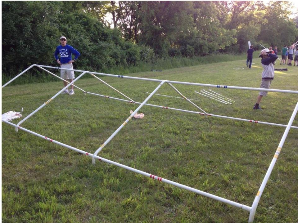
Assemble the canopy frame first, using the same color code for the corner pieces as for the poles. There is one set of unmarked poles/corners. These fit together as the “bare pair”. Assemble the legs and lay them around the roof frame at each corner and middle intersections.
